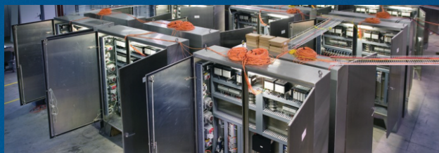
Houston, Tx: Facility, and fabrication yards
